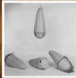
Blimp or zeppelin type one-bird container designed for use in releasing pigeons from high-speed planes. The propeller operates on a threaded swivel that opens the container to free the bird after being cleared from the wash of the plane.
